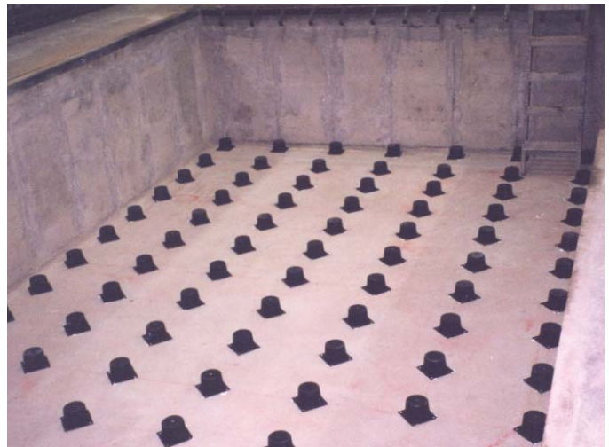
Type 2T Infab™ isolators positioned on pit floor prior to forming the foundation above.
