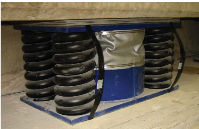
Coil spring isolator with integral viscous damping unit.
