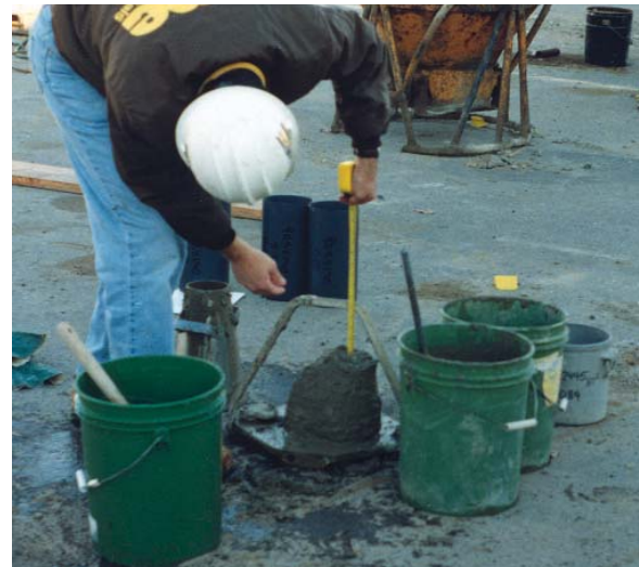
Concrete sample and slump measurement of concrete mix before pouring foundation.
