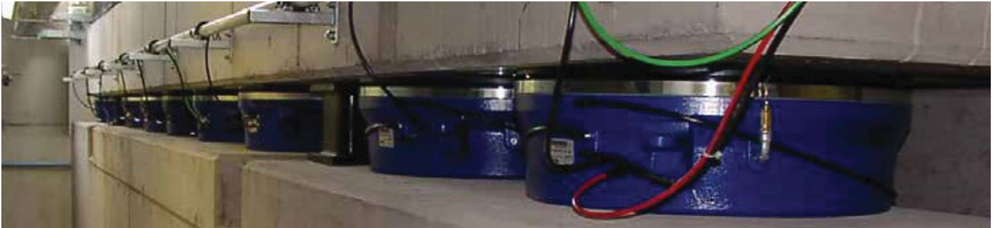
Fabreeka PAL type low frequency, pneumatic isolators support and isolate a foundation having moderate displacement.
