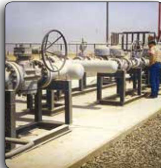
Client: Egyptian Natural Gas Co. Gas Pipeline Location: Egypt Valves: 12" Class 600 RF
